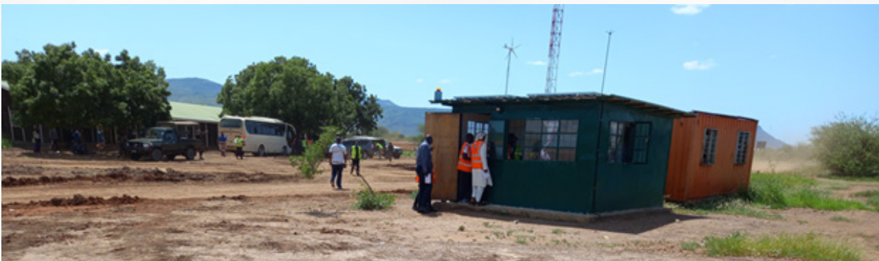
Foreground is the Kenya Immigration office at Nadapal. Clearance of travellers is automated.
