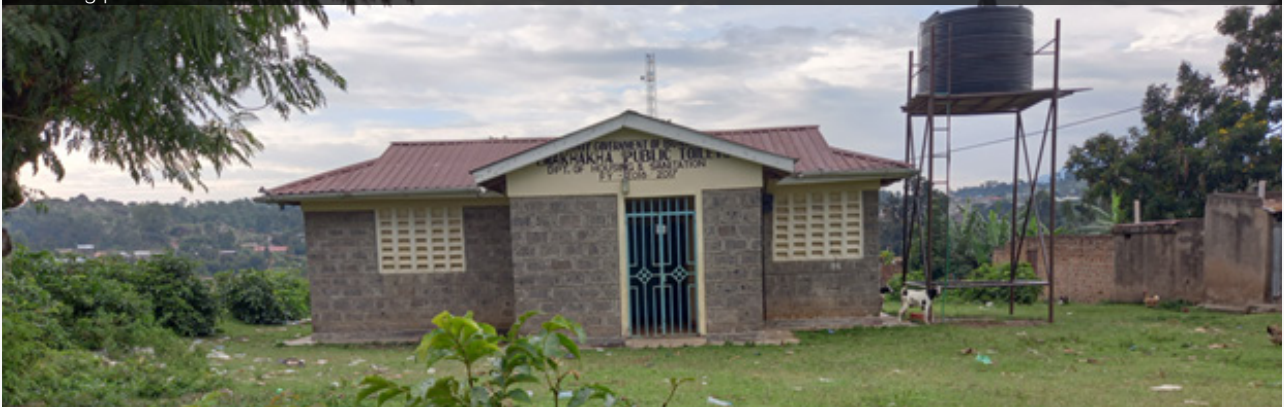
Below: The public facility is locked currently not available for use by the public. It is located very far (about 0.5Km) from the border crossing point and offices.
