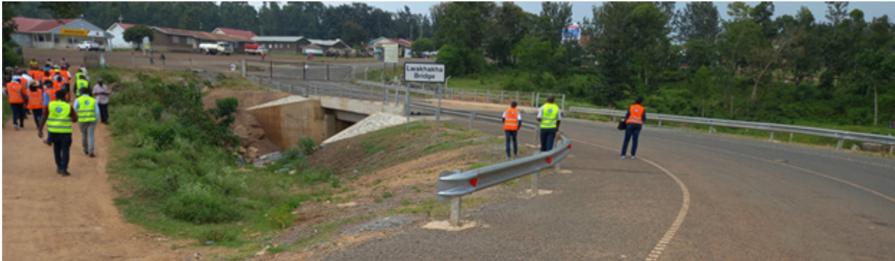
Above: Winding access roads to the Lwakhakha bridge raise safety concerns; potential risk of a heavy commercial vehicle colliding with another oncoming vehicle as they cross the border
