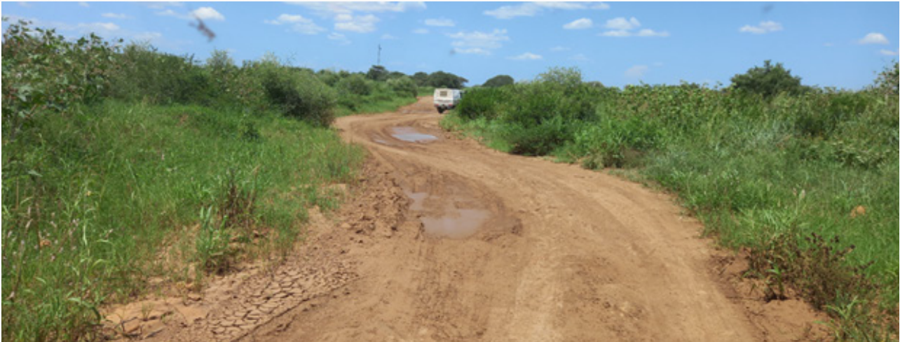
Section of the 1 Km stretch of road between Kenya and the South Sudan Government offices at Nadapal. When it rains, or they experience flash floods, the road is impassable, especially for trucks.
