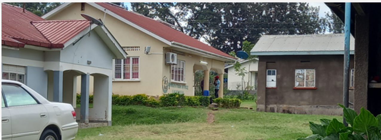
Uganda Immigration office at Lwakhakha. The office is hidden behind other buildings and not easily traceable by travellers. The immigration officers are also unable to see whoever is entering or leaving the country from the point where the office is located.
