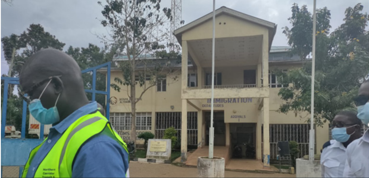
Above: Kenya – Lwakhakha Border Control Complex houses offices for Government agencies working at the border.
