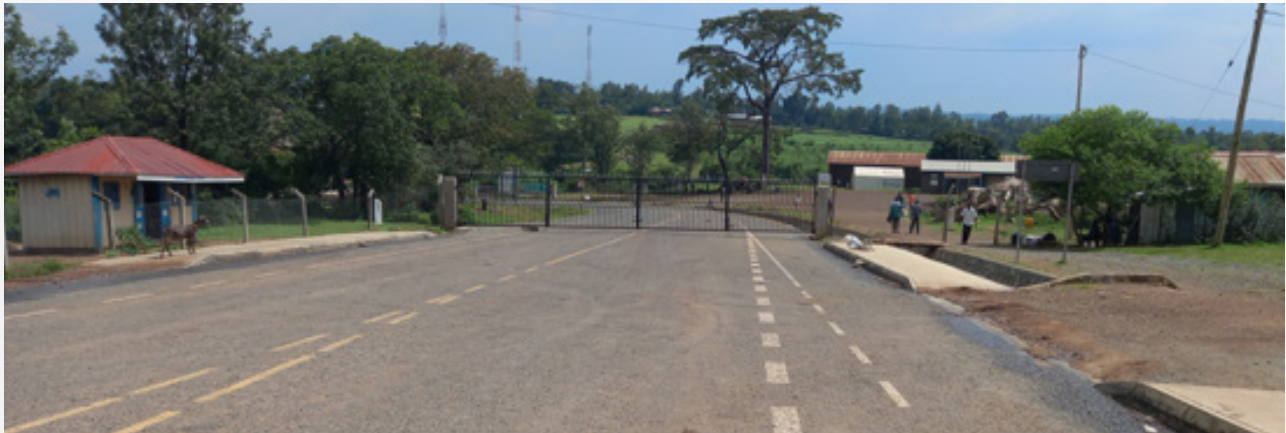
Above: Uganda side of Lwakhakha border station - Road from Lwakhakha border crossing point to Uganda. Uganda constructed a Class A dual carriage road over a km long with pedestrian walkways to facilitate the movement of motorists and pedestrians crossing the border.
