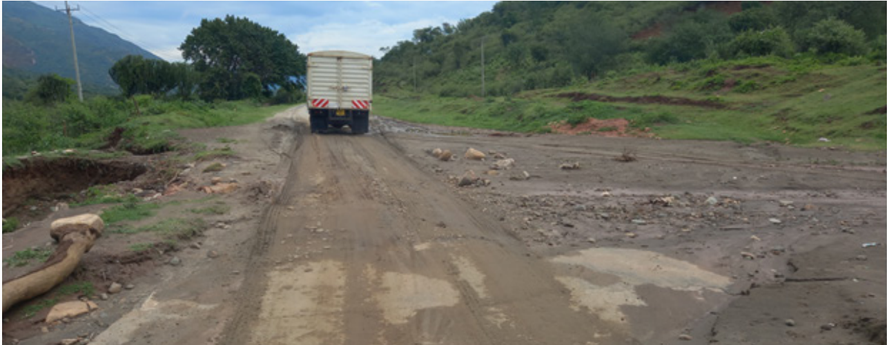
When it rains, the floods carry soil and rocks into the road, raising safety concerns for the road users.
