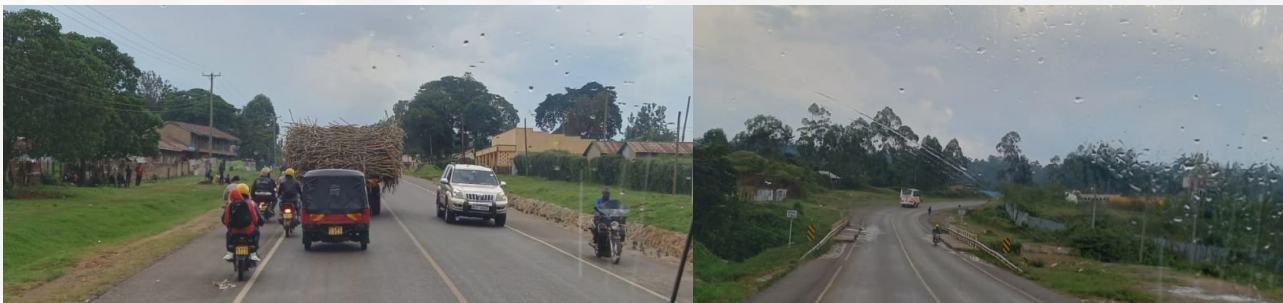
Left: Tractors transporting sugar canes obstruct the view of motorists behind them. Right: A black spot at narrowed carriageway at River Yala bridge located at Iguhu along the Kisumu – Webuye road. Should a tractor carrying sugar canes such as the one in the photo above meet at this bridge with a heavy commercial vehicle coming from the opposite direction, the likelihood of an accident is high.
