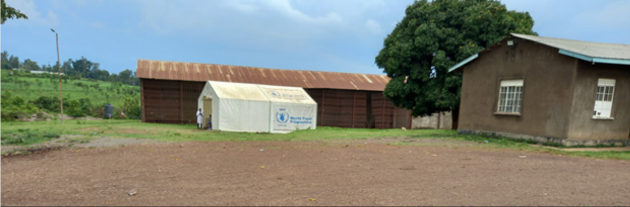
Behind the tent that serves as the Uganda Port Health office is a derelict customs warehouse that is not in use, and on the right, the old customs office is also not in use. It was observed that the structures not in use are occupying valuable space. Given the proposed plans for the Lwakhakha border station, it is not worthwhile to renovate these structures.
