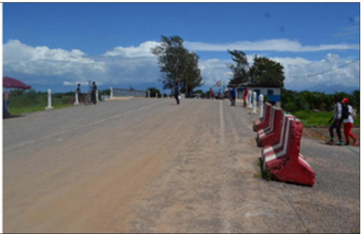
Right: December 2019, the capacity of the bridge has been upgraded to carry heavier loads with two lanes for motorized traffic and pedestrian lanes on each side.
