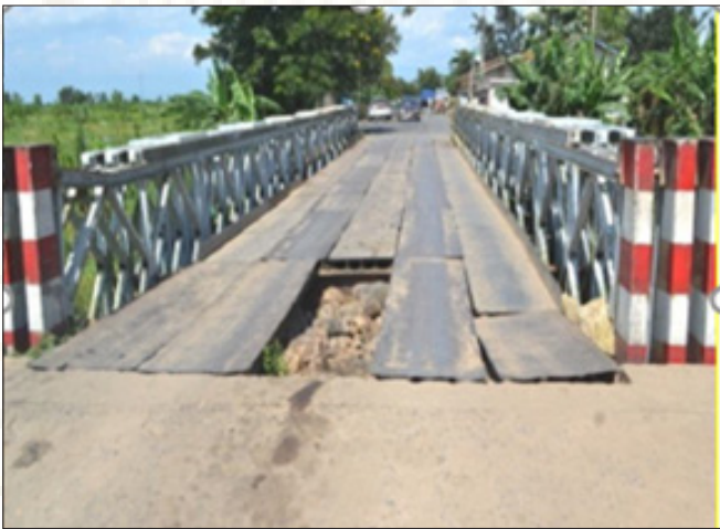
Left: March 2013, the single lane bridge without pedestrian walkway at Gatumba/Kavimvira border station at the Burundi-DRC border crossing point was in need of repair, NCTTCA survey team recommended upgrade to increase its capacity
