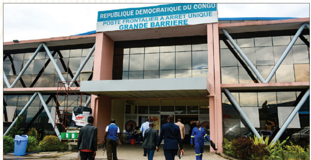
Below: December 2019, Grande Barriere OSBP offices at Goma – DRC/Rwanda border station.
