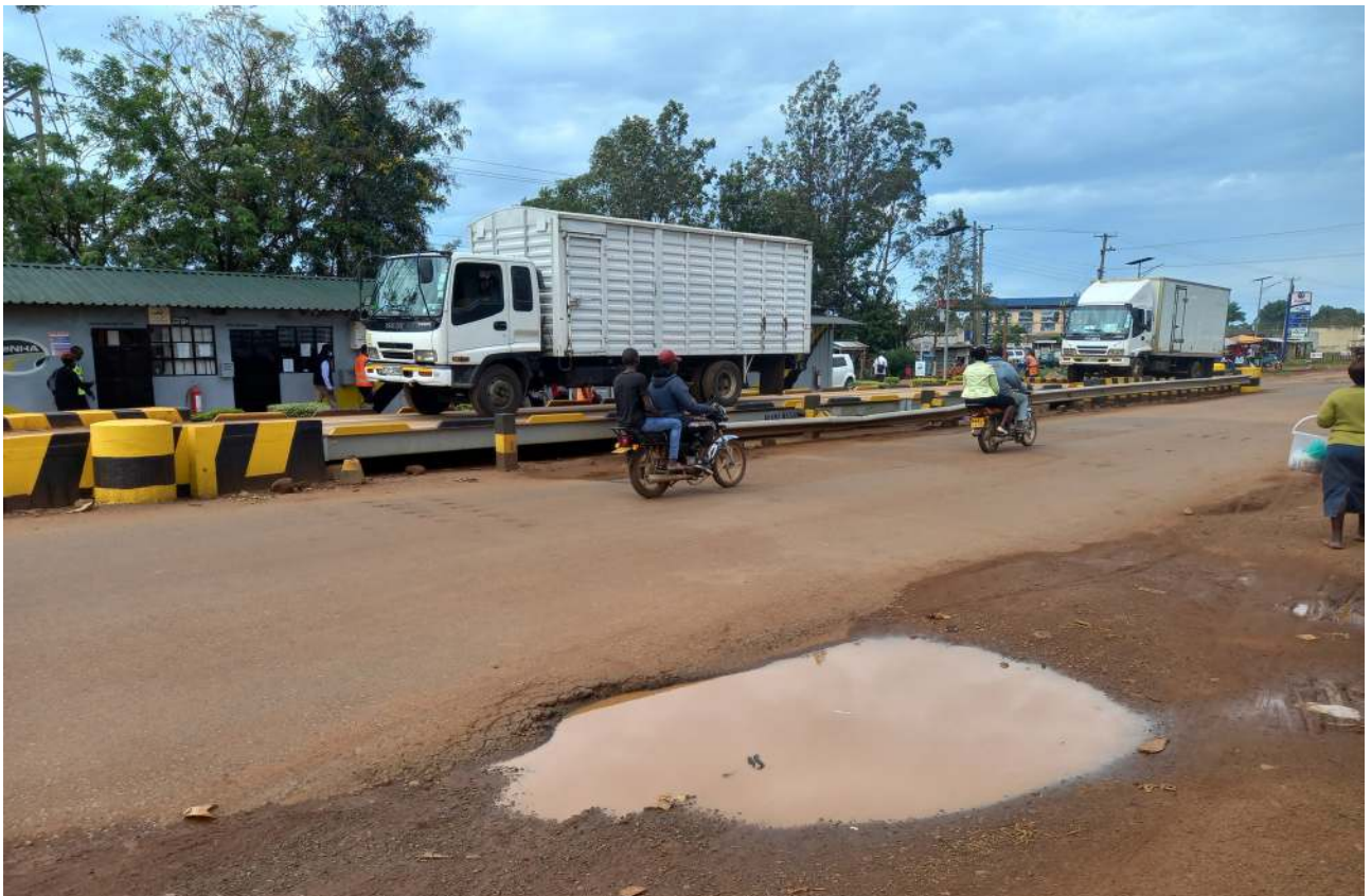
A truck is weighed at a static weighbridge in Kenya
