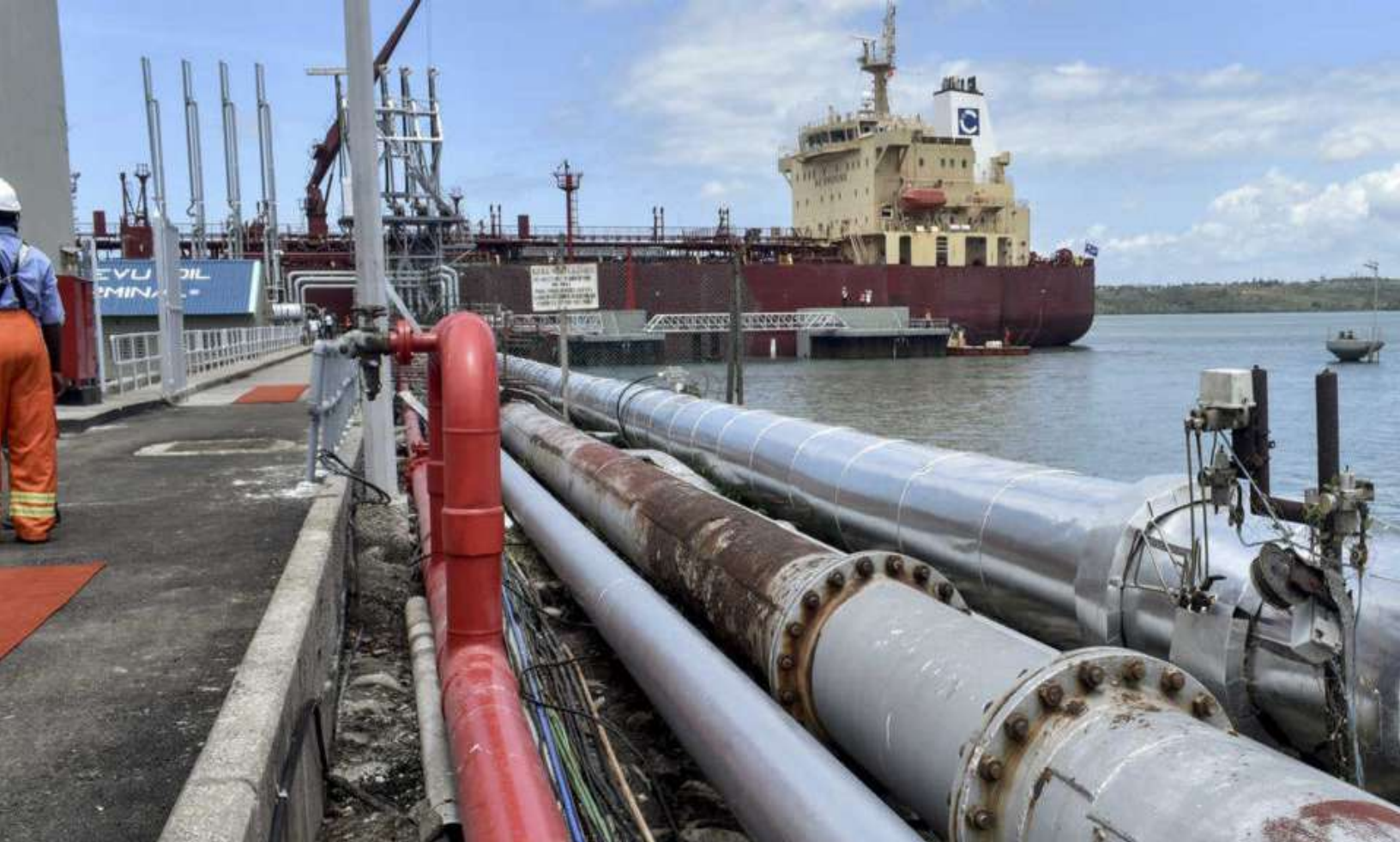
Kipevu Oil Terminal at the Port of Mombasa
