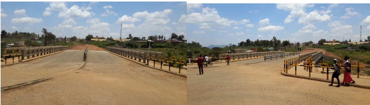
Left: The New Malaba Bridge; Construction of roads leading to the bridge on Kenya side was completed, Roads on Uganda side pending construction. Right: Pedestrians at the Kenya side have to cross over to the old bridge which has no pedestrian walkway because the access road on the Uganda side of the bridge is not yet completed. Benefits of the new bridge are not being realized, furthermore, it is contributing to the congestion at the border and high border crossing time.
