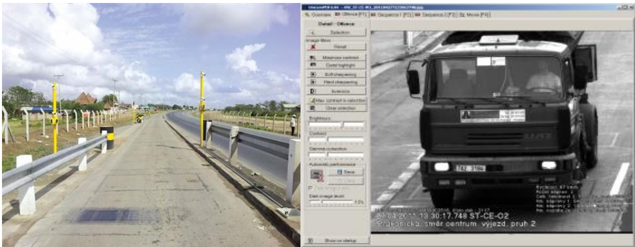
Left: Screener lane showing HSWIM loops and cameras Right: Traffic Data – all particulars of the truck including image are captured on computer and can be viewed from a remote screen such the one above.
