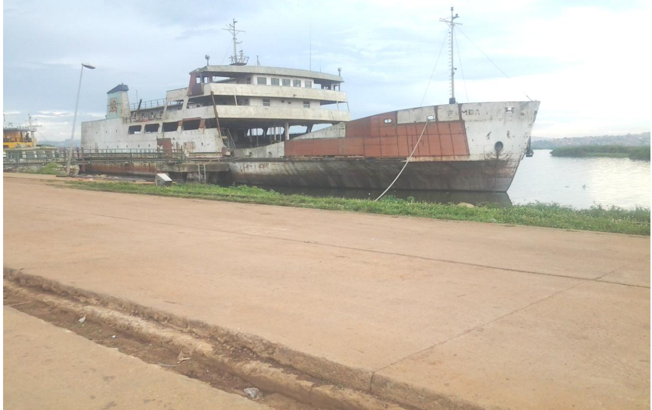
Refurbishment of MV Pamba is still pending. Efficient operation of wagon ferries is dependent on a well functioning railway system. MV Kaawa and MV Pamba have a capacity to carry 22 wagons i.e 44 TEU's.
