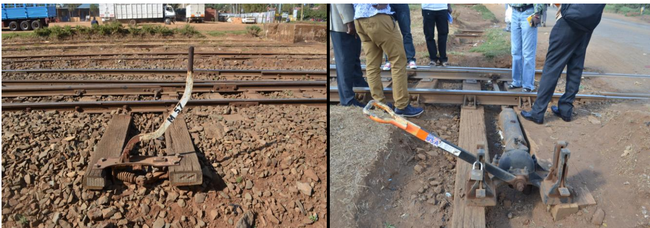
Left: Manual railway line interchange lever Right: Automated railway line interchange lever
