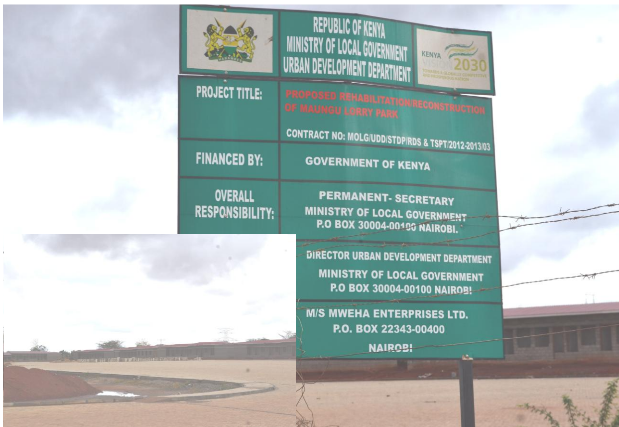
Inset: Maungu Lorry Park under Construction
