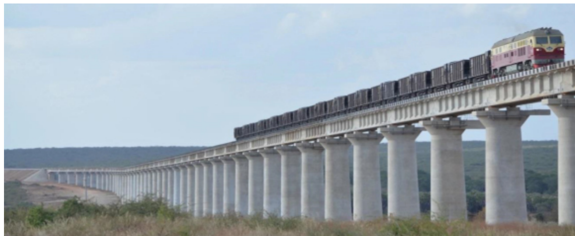
A completed section of the SGR track between Mombasa and Nairobi
