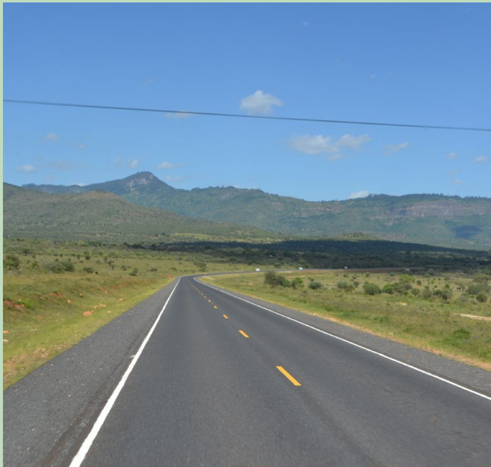
A section of Voi- Holili road
